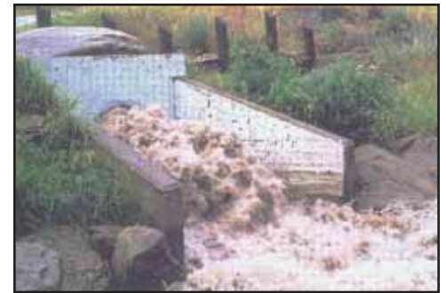
June 2005: Stormwater outfall
